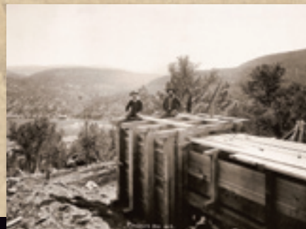
Example of the pressure box used on the Hanging Flume.
