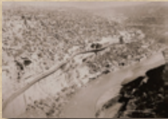
Aerial view of the completed flume. Photo by W.J. Carpenter
