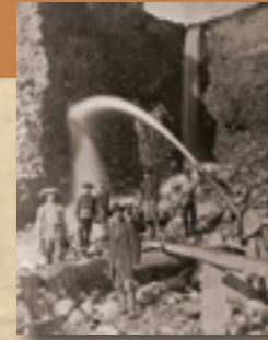
Example of placer mining. Taken in California.
